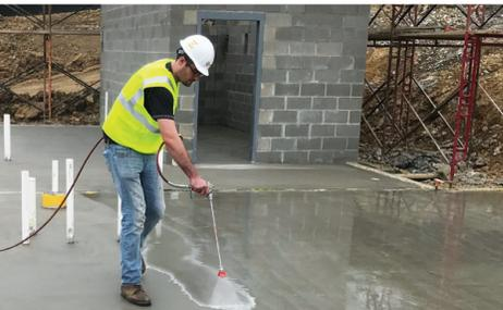
days during the winter months, longer set times could push SCP product application to a later time when temperatures are too cold. Application may need to take place the following morning. If this is the case, the concrete company may need to protect the concrete with blankets or other means.
