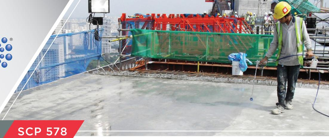
**SCP 578** is a penetrating colloidal silica concrete treatment that is spray-applied on existing concrete. SCP 578 is a permanent alternative to traditional moisture mitigation systems.
